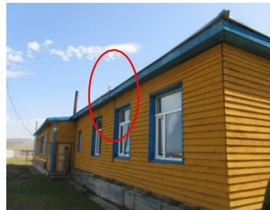
WiFi Antenna at Hospital
