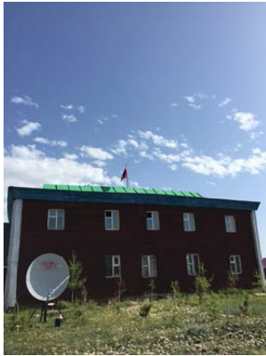
VSAT Antenna in front of Local Government Office
