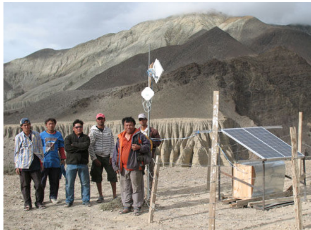
Relay Station in Kagbeni
