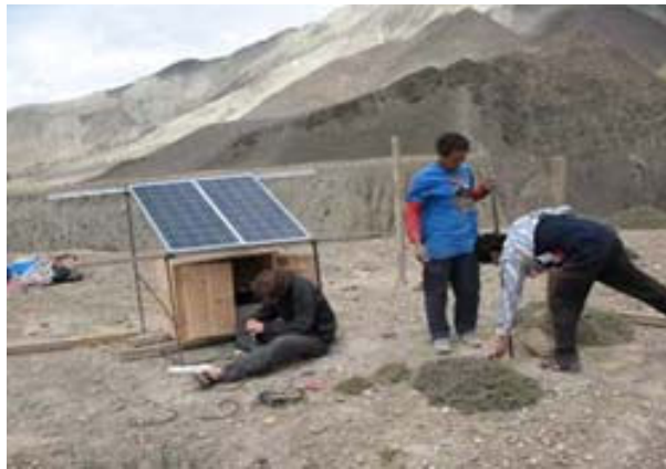
Building Relay Station in Kagbeni
