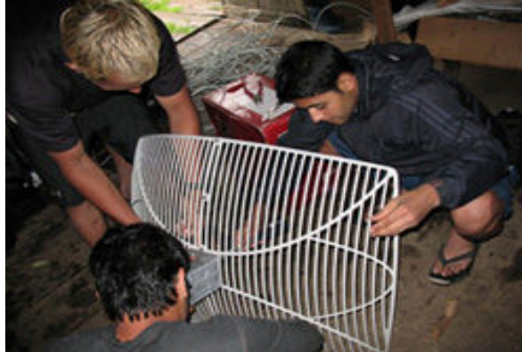
Assembling Grid Antenna at Mohare Relay
