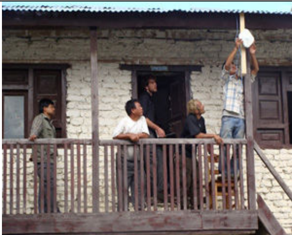
Installing Client radio at Tukuhe School
