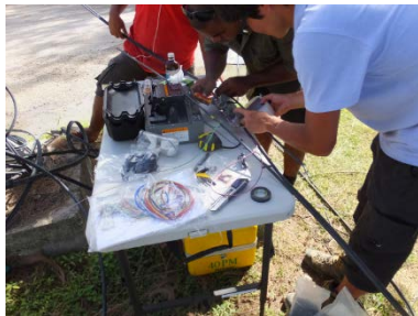
Fusion splice at the field practice taught by OCC engineer (1 st time in Nauru)
