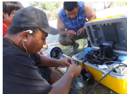
Learning how to make fusion splice with fibers, at the room and field
