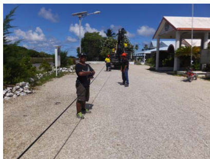
Pull the optical fiber cable by pickup truck
