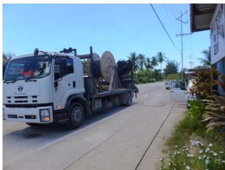
Roll down the cable
