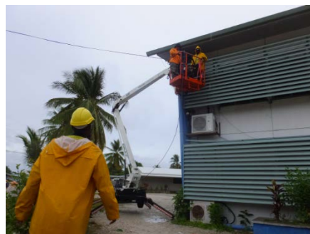
Fiber cable into building in rain
