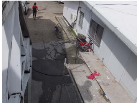
Laying the optical fiber cable among buildings
