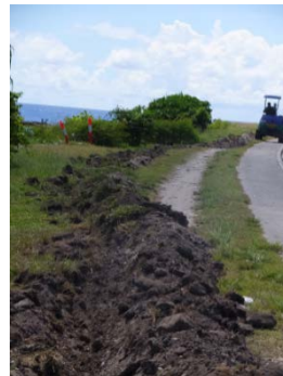
Digging and laid the optical fiber cable but not whole route.
