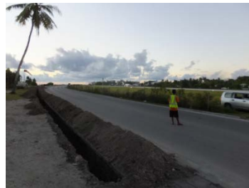
Digging and laid the optical fiber cable but not whole route.
