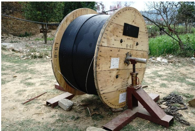
Figure 39: Cable Drum mounted on Tripod Jack
