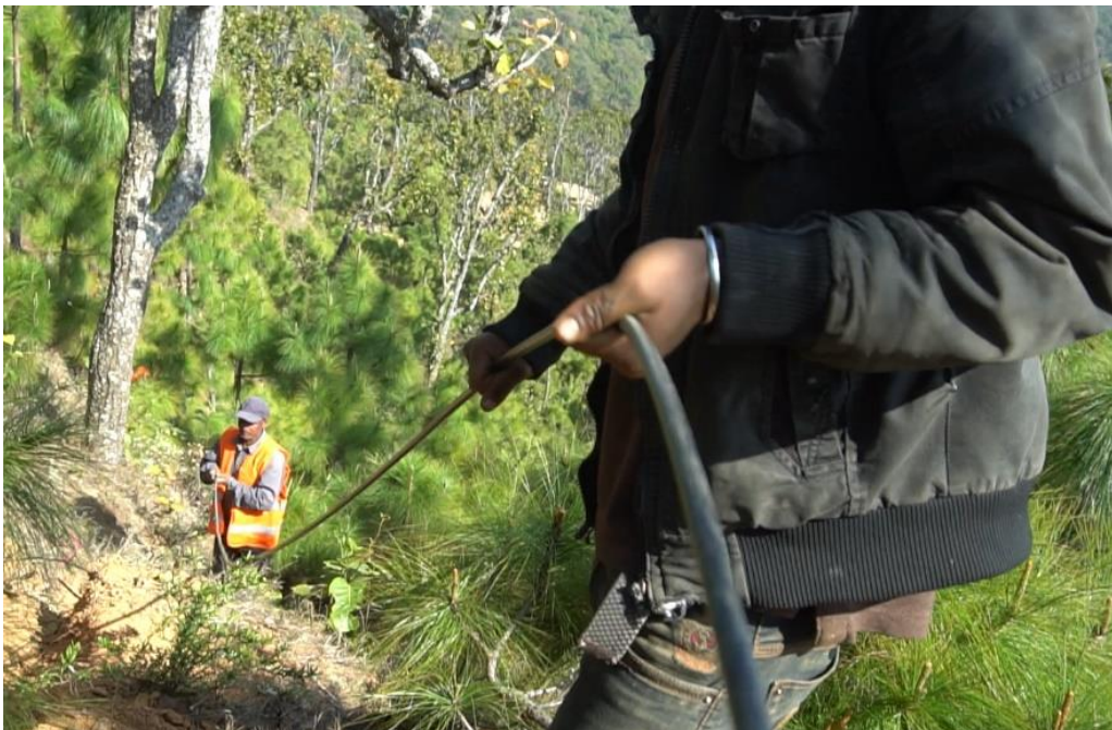
Figure 9: OFC (F-PAC) Laying in Jungle Terrain
