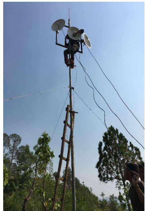
Figure 40: Wireless Antenna Install on Repeater Station at Rithha Farmer's Private Land
