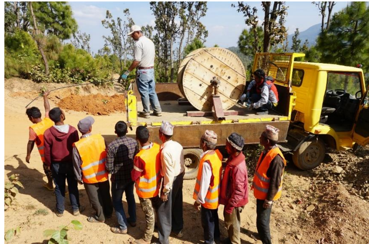
Figure 42: Optical Fiber Cable unrolling by pickup and training of Dullu residents
