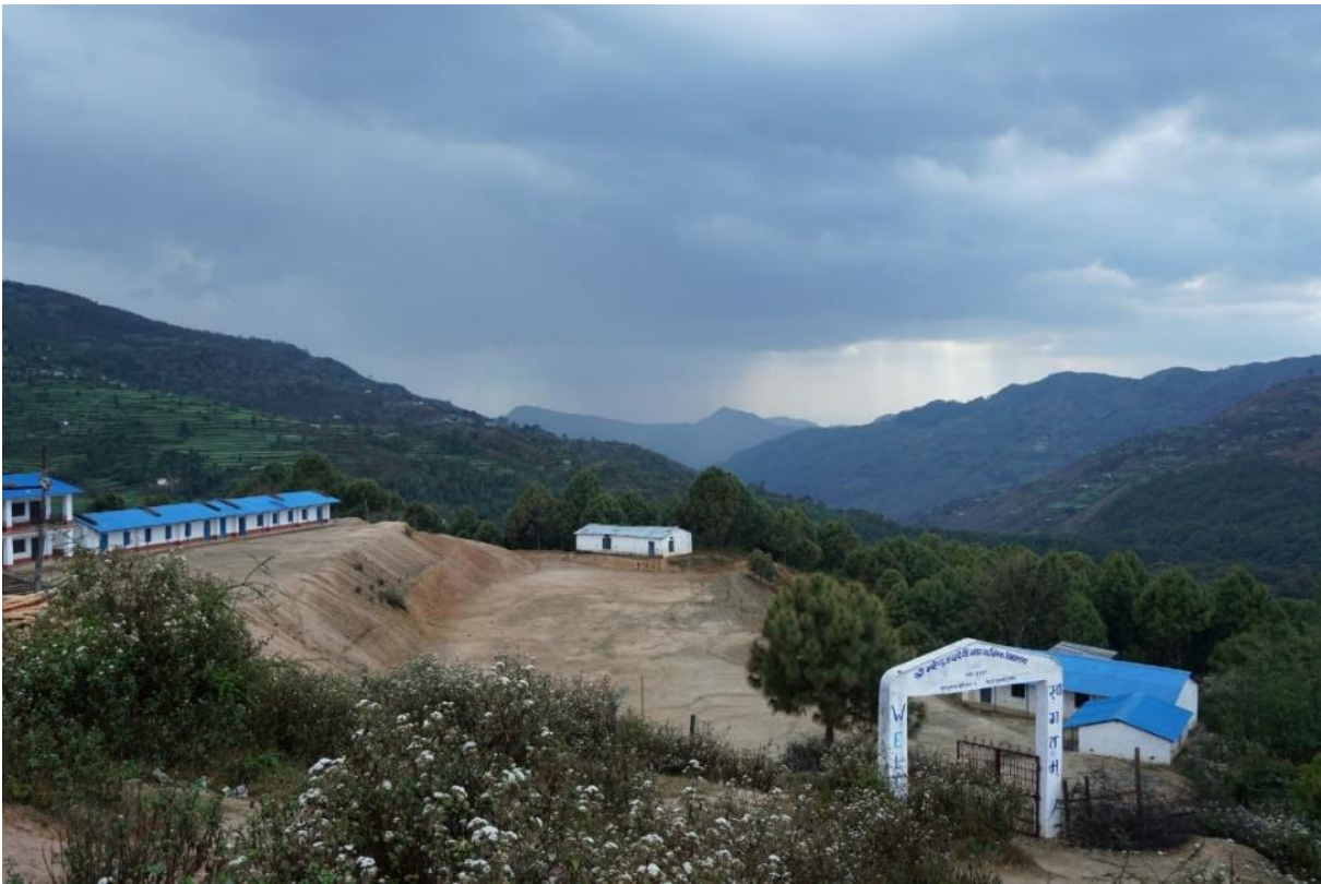
Figure 36: Dullu Municipality High School near Ward 6 (OFC Start Point)
