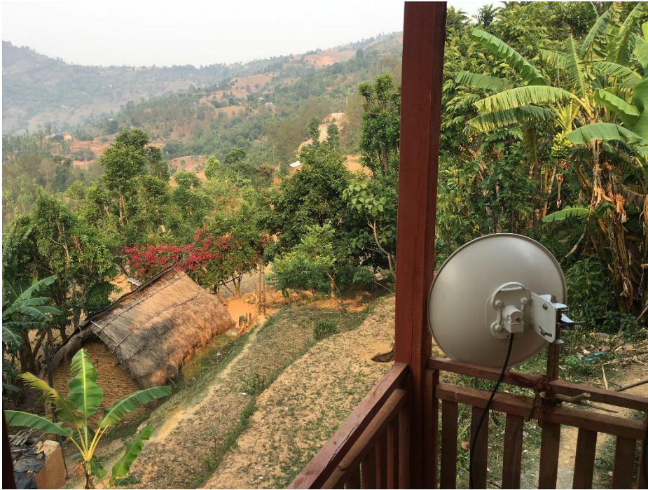
Figure 30: Dullu Municipality Ward 9 Wireless Antenna P2P Link
