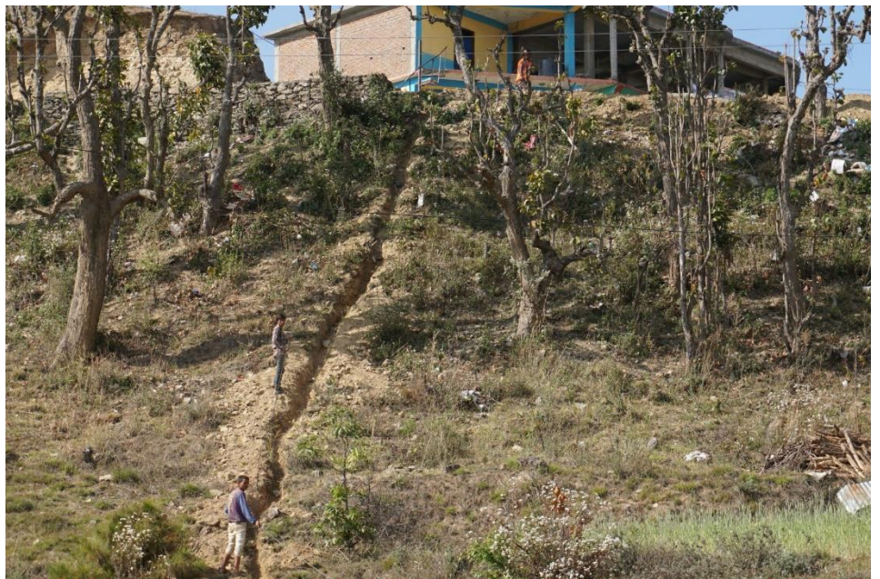
Figure 26: Optical Fiber Laying along Hilly Terrain
