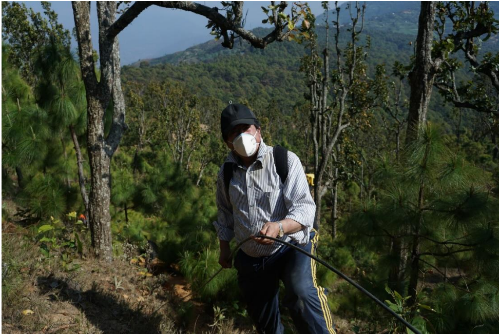
Figure 28: Dr. Okamura Laying OFC in Jungle and Hilly Terrain
