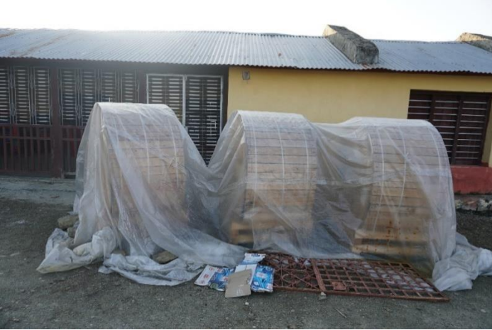
Figure 44: Dullu Municipality Storage of Cable Drums
