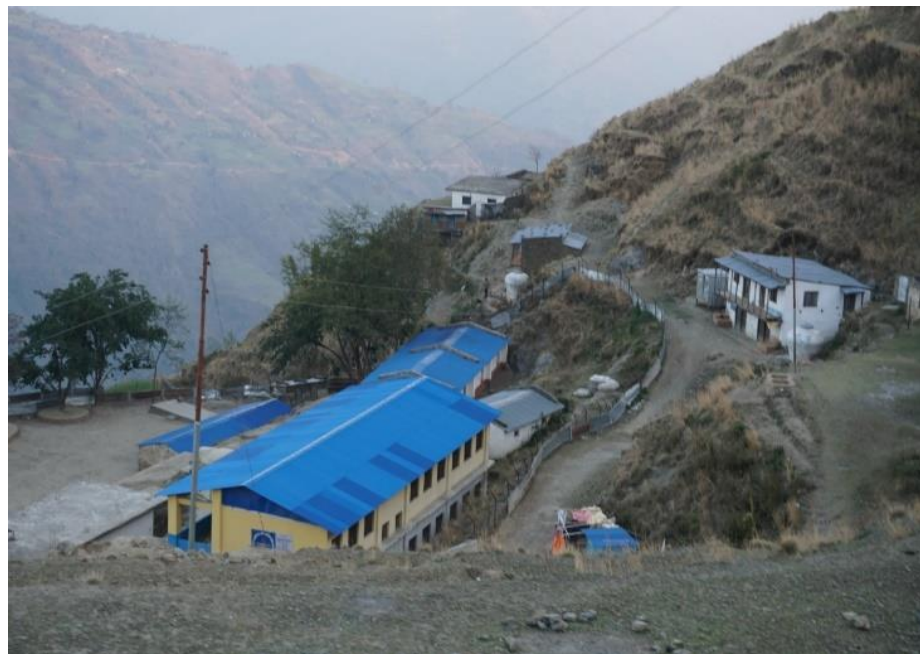
Figure 37: Dullu Municipality Ward 11 School and Health Post
