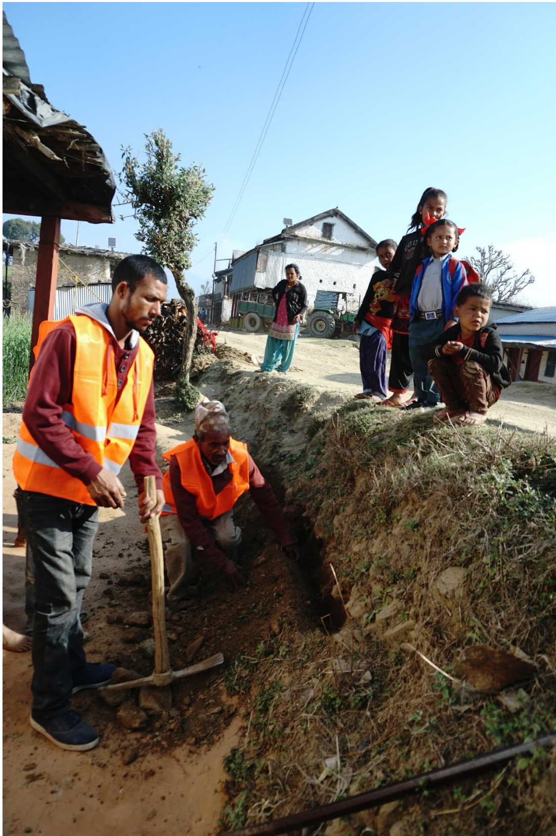
Figure 33: OFC Layout on 'cliff' side of a raised road
