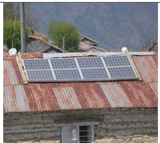
Solar panel Installation in Tikot village
