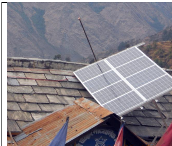
Solar Panel Installation in Paudwar village
